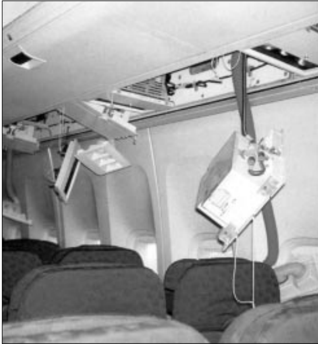
Three passengers said that they were struck by passenger service units that dislodged during the accident. (Photo: Australian Transport Safety Bureau)
