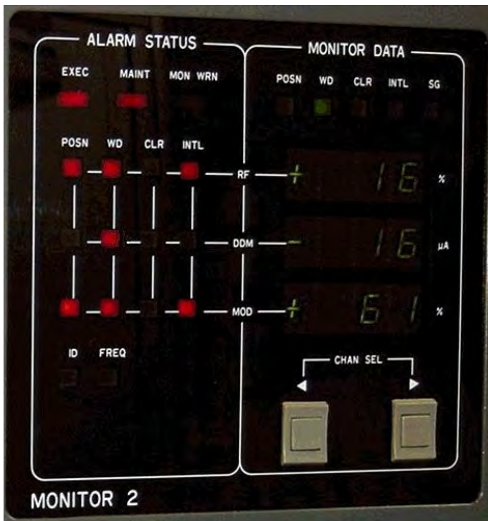
Close up of one monitor panel
